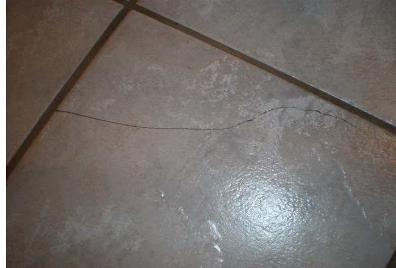
807. Cracked Floor Tiles
