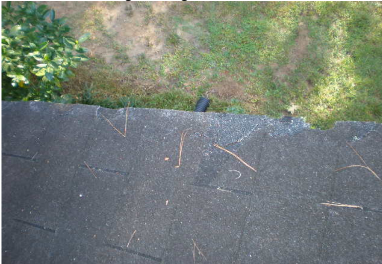
312. Cracked/Damaged Shingles
