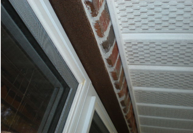
213. Exterior Wood Rot/Decay
