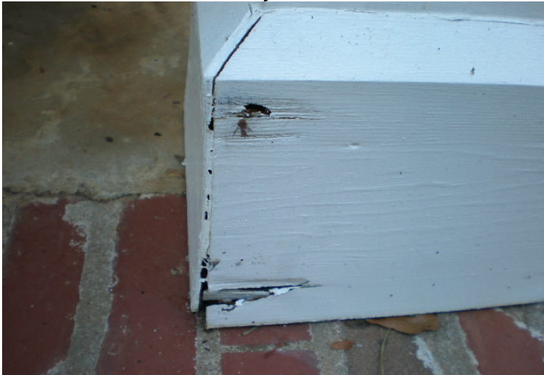
213. Exterior Wood Rot/Decay
