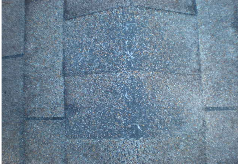
312. Cracked/Damaged Shingles
