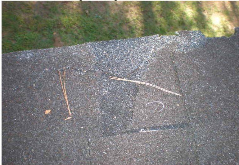
312. Cracked/Damaged Shingles
