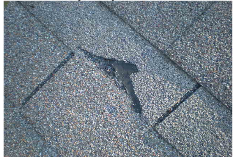
312. Cracked/Damaged Shingles
