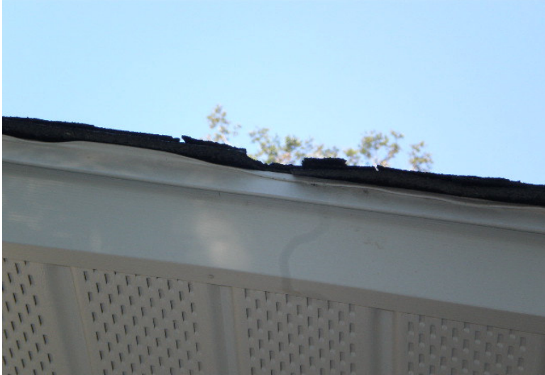
312. Cracked/Damaged Shingles
